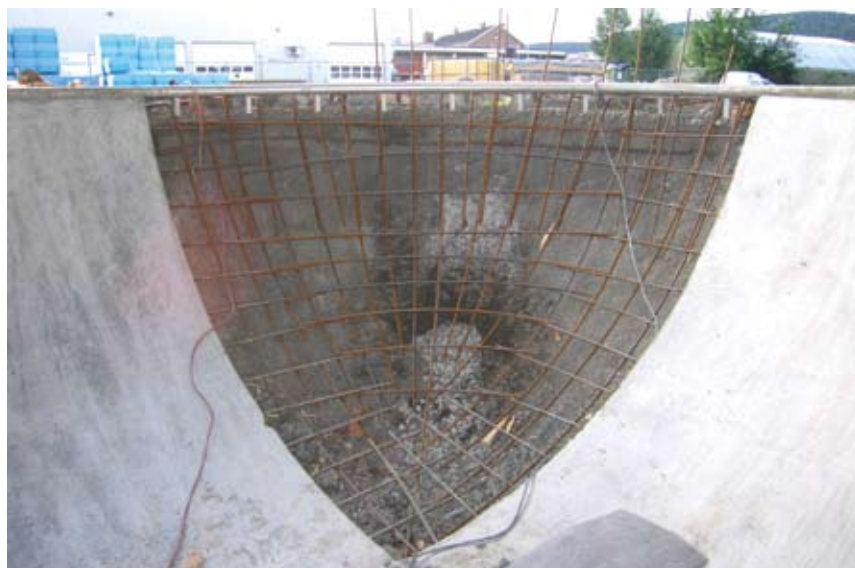
Ferdig armert felt i bowlanlegg
