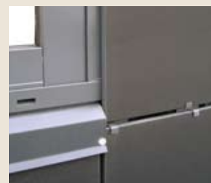
Figur 5d: Overgang vinduskarm/flisflate
