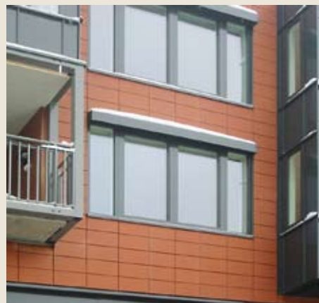
Figur 5d: Overgang vinduskarm/flisflate
